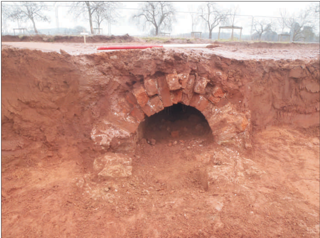
Plate 2: Culvert F107, viewed from the northwest. 1m scale
