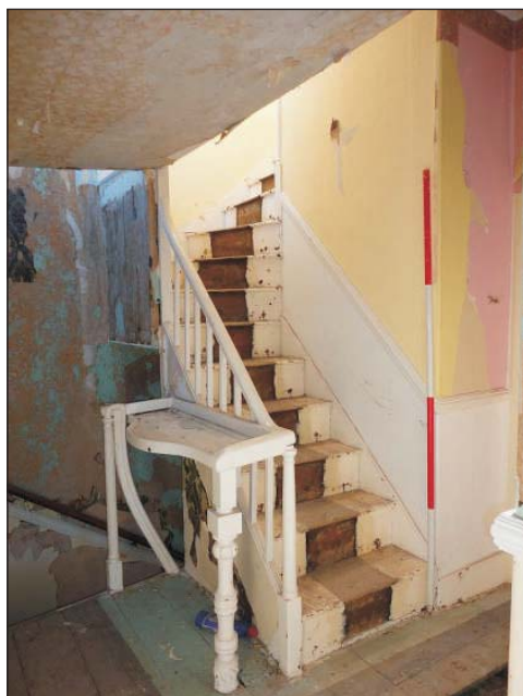
Plate 9: Detail of the staircase from the first-floor landing. Scale 2m
