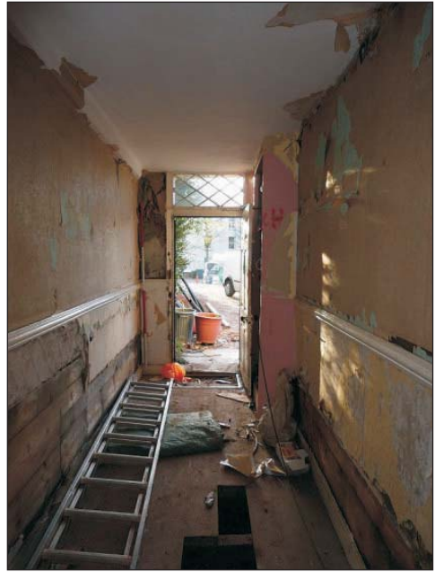
Plate 6: View of the passage showing boarded treatment below the dado. Scale 2m
