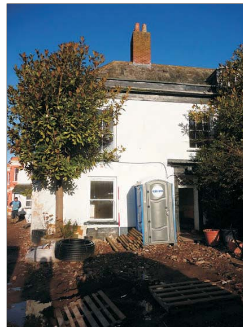
Plate 4: Detail of the front elevation of Magnolia House. Scale 2m
