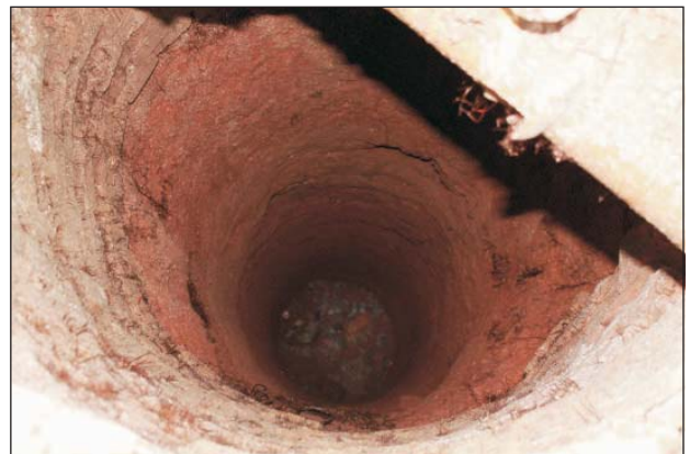
Plate 25: Well 1000 behind the Acacia House annex showing the lower courses of brickwork.
