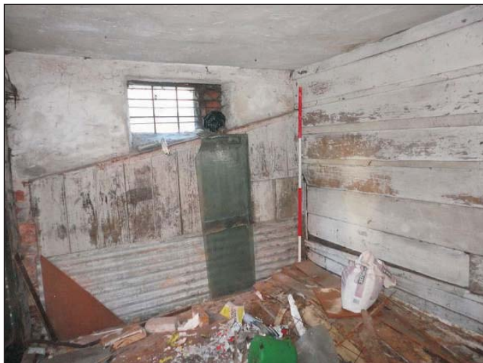
Plate 13: Detail of the surviving stallwork in the stable. Scale 2m
