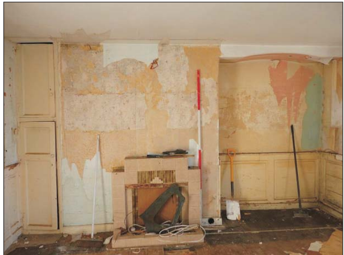
Plate 8: View of the northeastern wall of the parlour showing the panelling and fireplace after stripping out. Scale 2m
