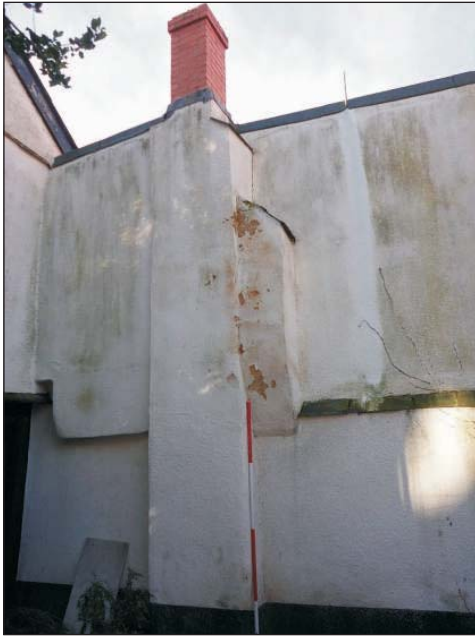
Plate 17: View of the rear wall of the annexe showing jettying and recessed features. Scale 2m
