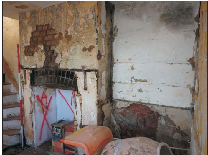
Plate 18: View of the larger ground-floor room in the annexe showing a 19th-century brick fireplace built against an earlier wall constructed of large blocks of breccia. Scale 2m
