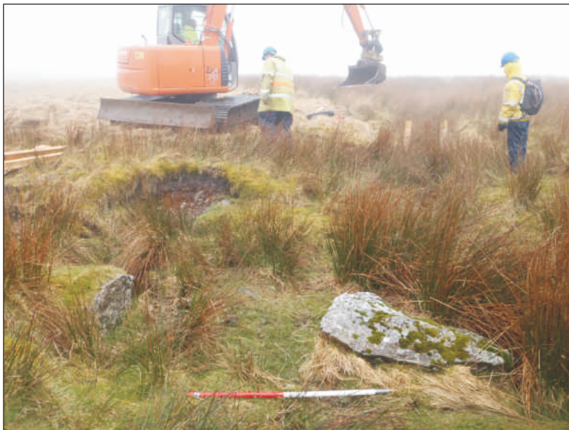
Plate 3: Intersection of ditches 6j and 7a showing large stones, viewed from the east (1m scale)
