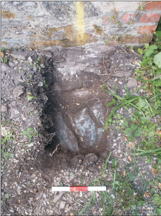
Plate 1: Possible surface F303 in pit 3, viewed from the east. 0.30m scale
