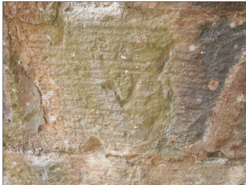
Plate 13: View of masons' mark under the bridge arch, taken from the south
