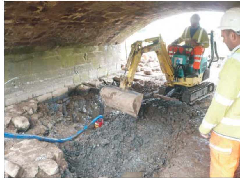
Plate 2: Working shot showing repair 104 in foreground, taken from the northeast
