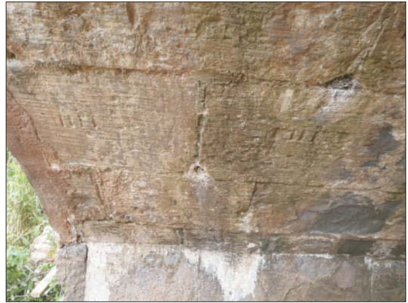
Plate 12: View of masons' marks under the bridge arch, taken from the south
