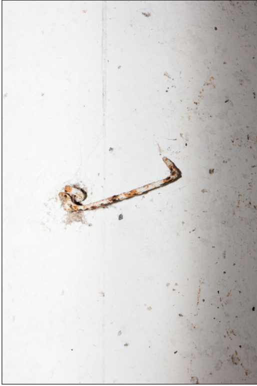
Plate 8: A securing hook for a window shutter, viewed from the south.
