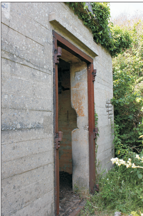
Plate 6: A doorway at Oxwich Bay showing the concrete hood, viewed from the southeast. Photo: Andrew Passmore.
