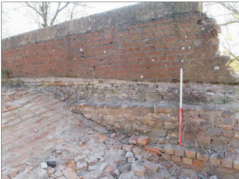
Plate 2: Close-up view of the bridge showing the brick arch and stone and brick face and parapet, viewed from the northwest. 1m scale.
