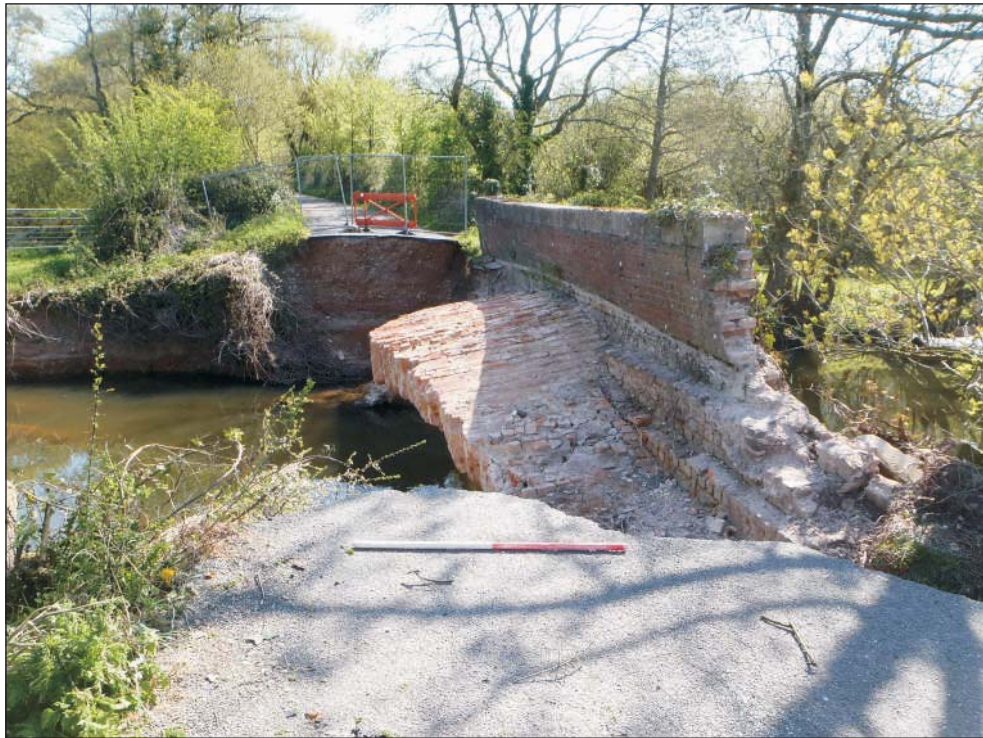
Plate 1: The collapsed bridge prior to demolition, viewed from the west. 1m scale.
