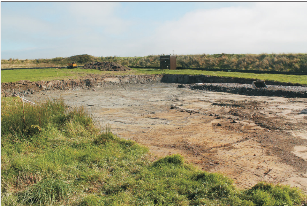
Plate 2: General view of the site taken from the northwest.
