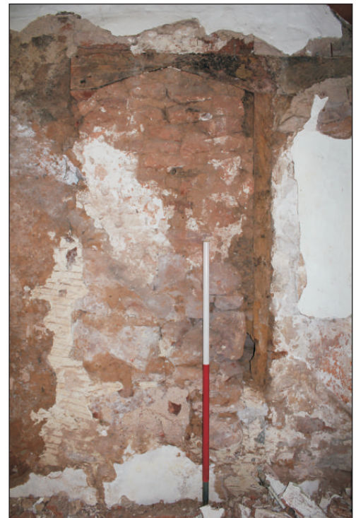
Plate 5: The southern of the two blocked doorways, viewed from the northeast. 1m scale.
