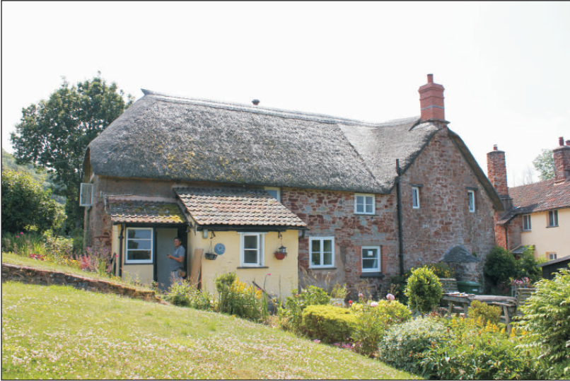
Plate 1: The front elevation of the house viewed from the north, showing the bathroom extension (painted yellow) with the hall, blocked cross passage and gable of the south wing beyond.
