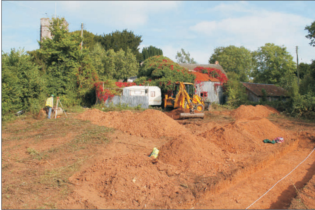
Plate 1: General view of site, looking east
