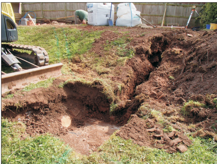
Plate 6: Concrete pad 116. View from the NW.
