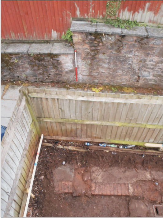
Plate 4: Alignment of N-S wall F106 with faced stonework in the retaining wall of the alleyway. View from the N (scale 1m)
