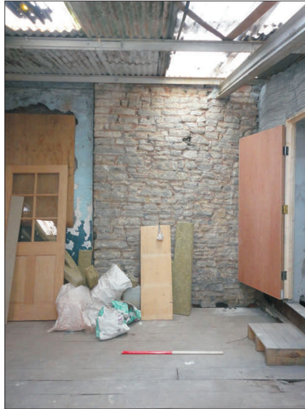
Plate 10: View within the rear wing showing the original rubble masonry of the side wall of No. 37 Stokes Croft (scale 1m)
