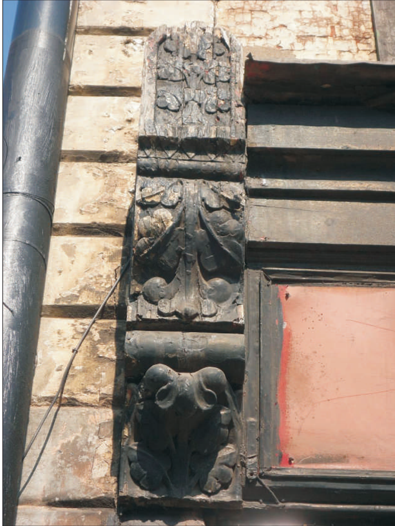
Plate 5: Detail of the ornamental corbel at the south-western side of the shop front, showing vigorous 19th-century foliage carving
