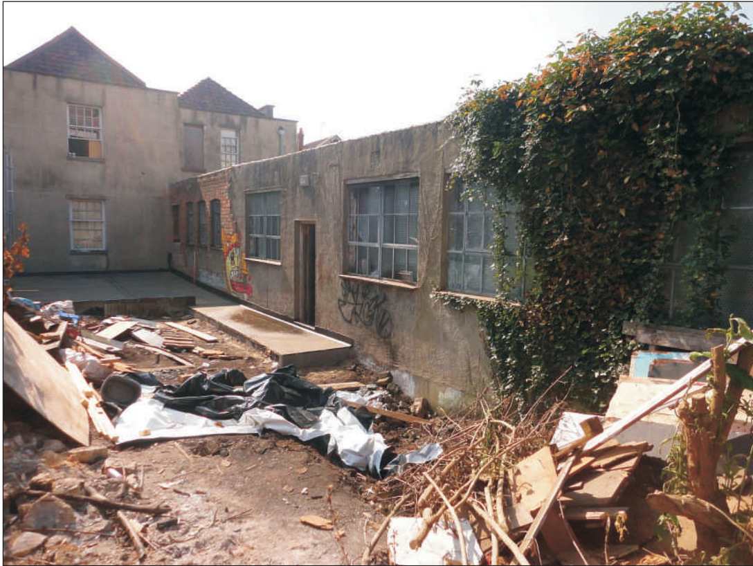
Plate 7: View of the rear of the buildings from the site of the proposed mews houses
