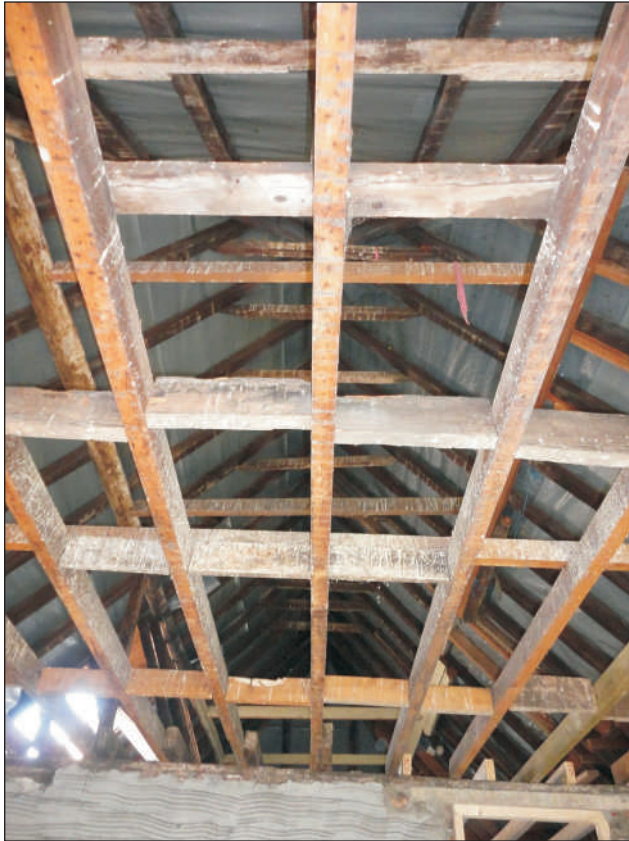
Plate 9: View of the 18th-century roof structure of No. 37 Stokes Croft showing traces of lath and plaster ceiling the attic rooms and (top) a chamfered trimmer for the original front dormer
