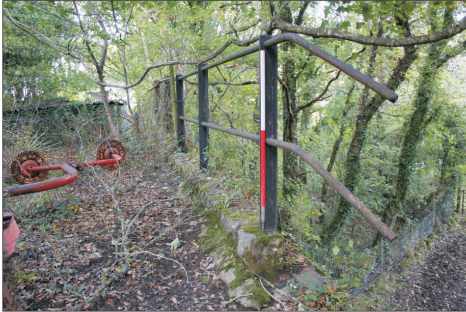
Plate 7: The parapet and railing, viewed from the south. 1m scale.
