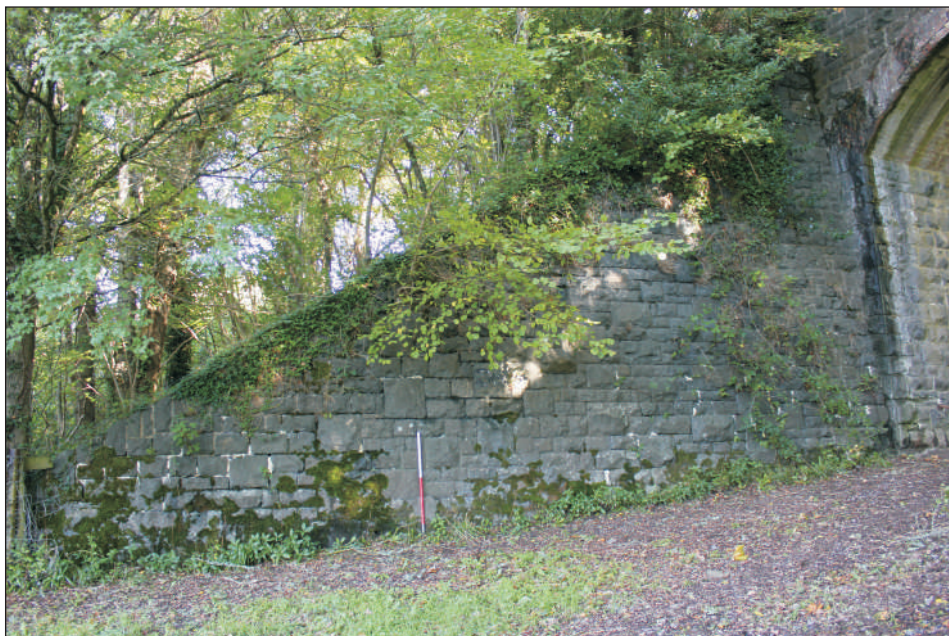
Plate 6: The west side north abutment, viewed from the south. 1m scale.
