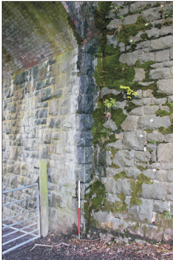
Plate 4: The east elevation showing quoins and separate abutment, viewed from the southeast. 1m scale.
