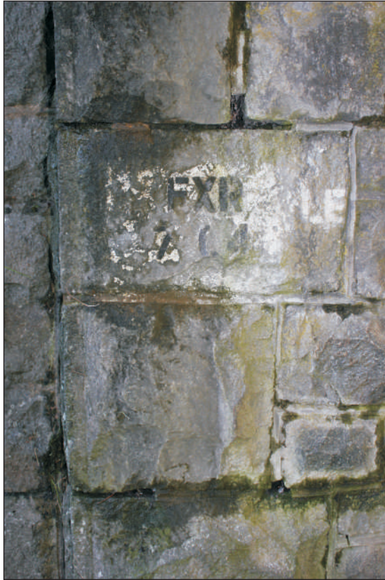
Plate 5: The sign, also showing a feather and tare hole on the stone, viewed from the south.
