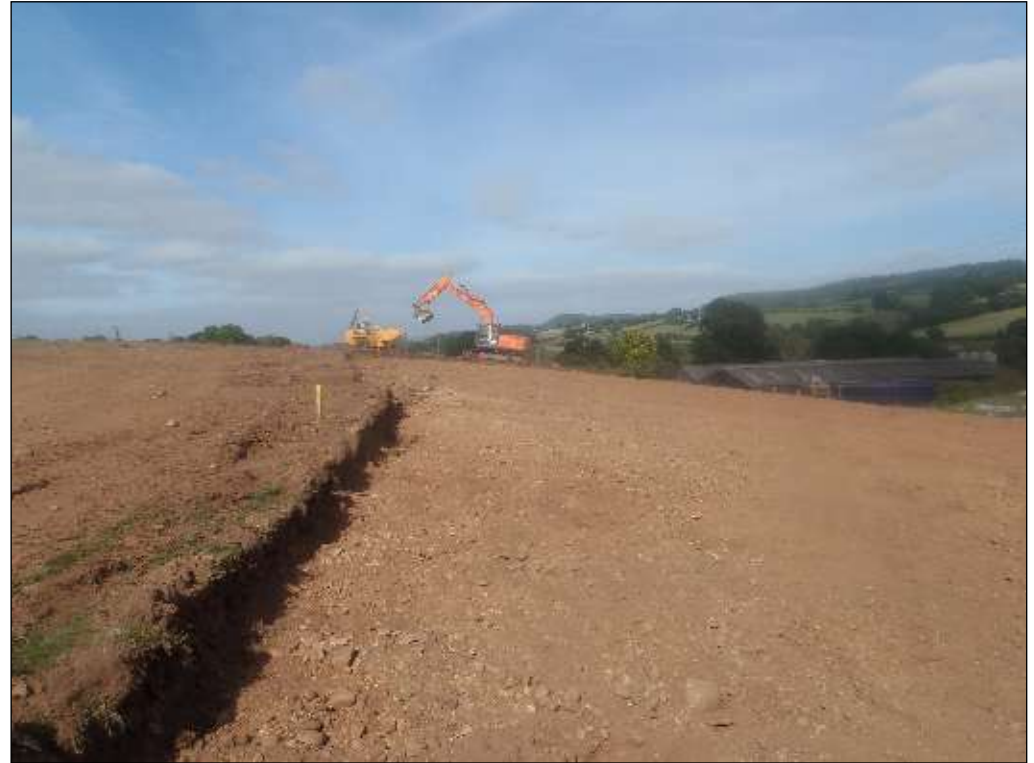
Plate 7: Area strip for new stock building, view from the west
