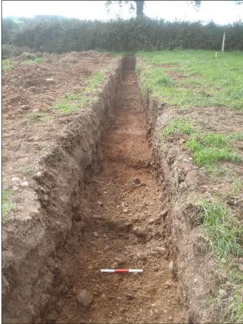
Plate 6: Linear features F176 and F178 within cable trench view from the north. Scale 0.3m
