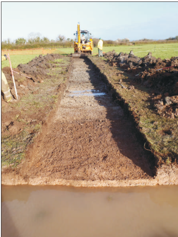
Plate 3: Trench 2, work in progress, viewed from the southwest
