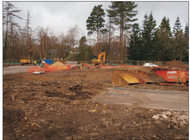
Plate 4: View of the residential development area, looking northwest
