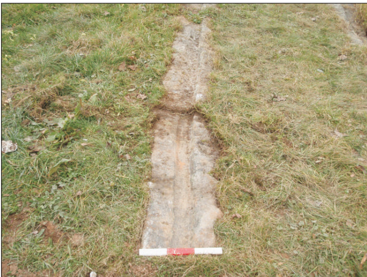
Plate 7: Detail of southwest line of the Haytor Granite Tramway, looking northwest (scale 0.3m)
