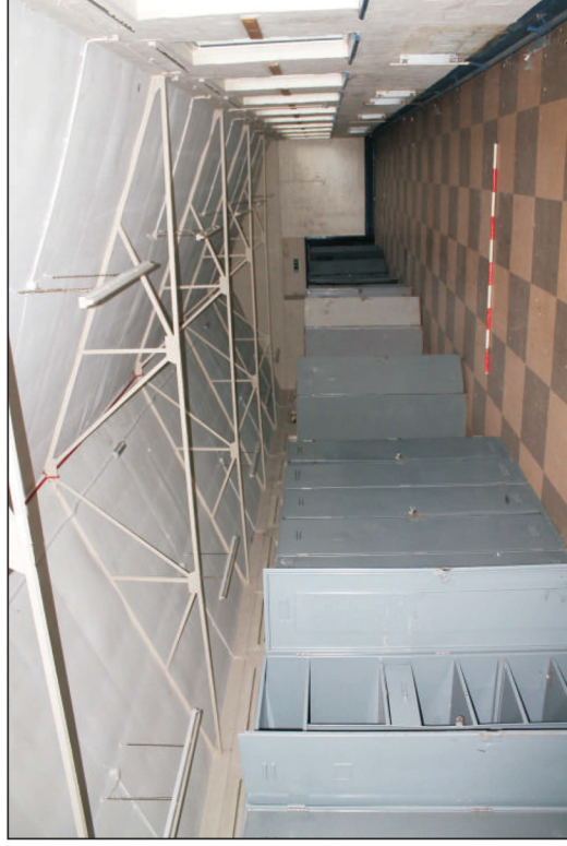
Plate 12: Building 7, ward showing open-plan ward and exposed roof truss viewed from the south. 2m scale
