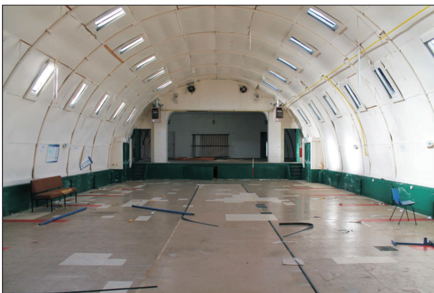
Plate 23: Building 35, Mountbatten Hall, interior viewed from the northwest. 1m scale
