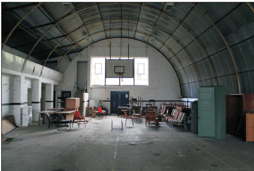
Plate 21: Building 77, The Ship, interior showing raised viewing platform to left, viewed from the west. 1m scale
