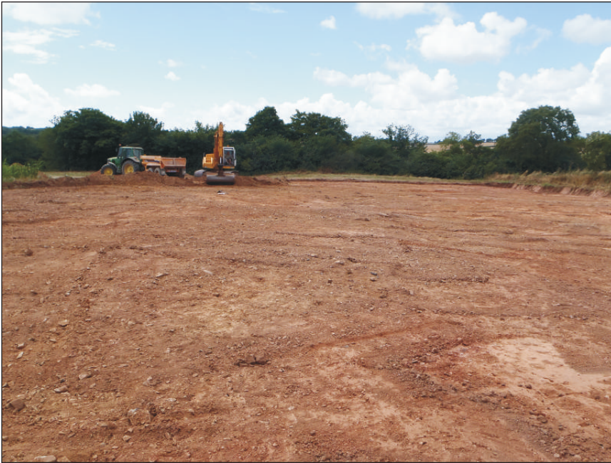
Plate 1: Topsoil stripping, looking southwest
