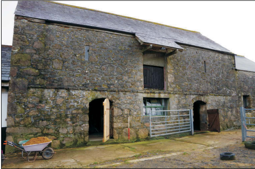
Plate 1: Room B, viewed from the south. 1m scale.
