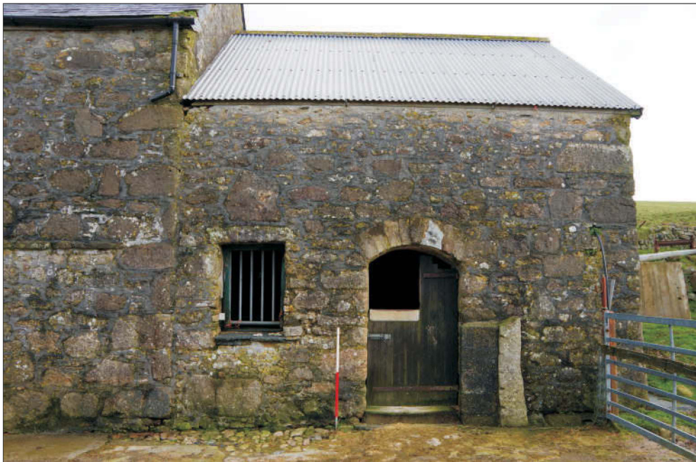
Plate 2: Room C, viewed from the south. 1m scale.
