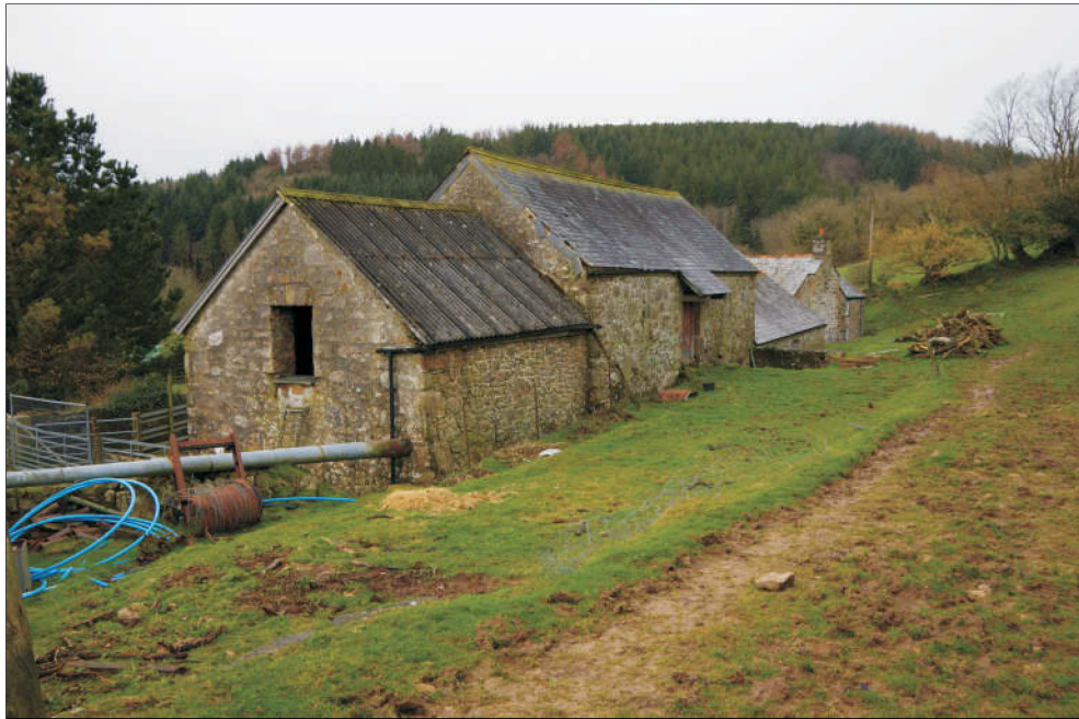
Plate. 5 The building viewed from the northeast, showing the rear elevation and the east elevation of room C.
