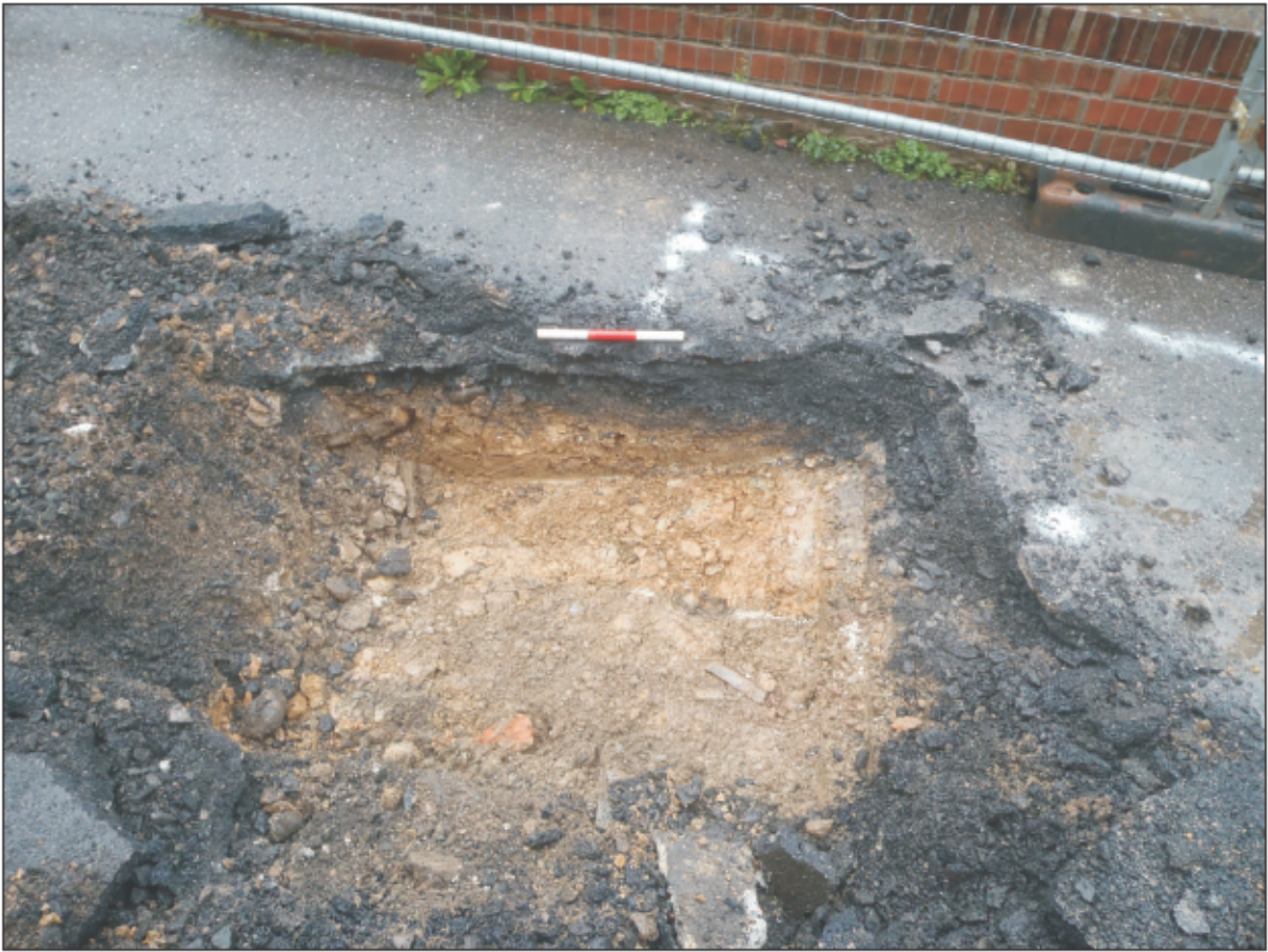
Plate 1: Tree pit 1, viewed from the west (0.3m scale)
