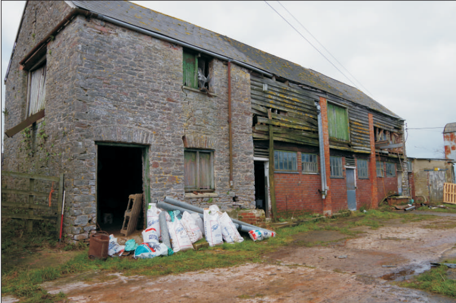
Plate 7: Building 3, southeast and northeast elevations, viewed from the southeast. 1m scale.
