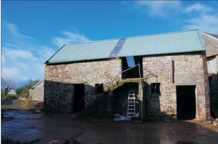
Plate 10: Building 4, southeast elevation showing alterations, viewed from the southeast. 1m scale.
