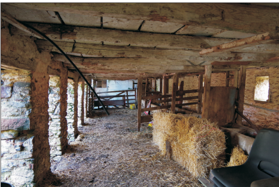
Plate 6: Building 2, interior, viewed from the southeast.
