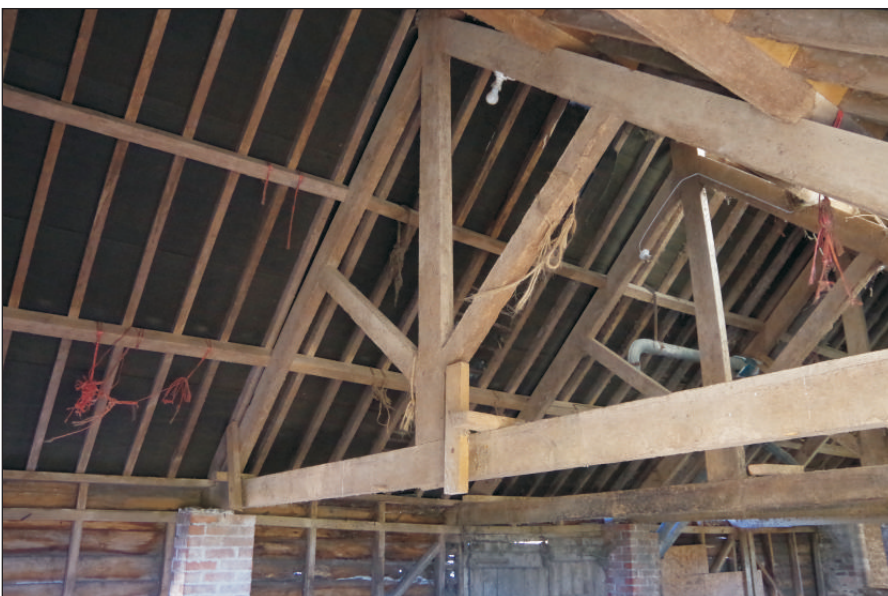
Plate 9: Building 3, the roof structure, viewed from the northwest.
