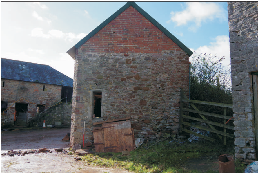
Plate 11: Building 4, northeast elevation showing alterations, viewed from the northeast. 1m scale.
