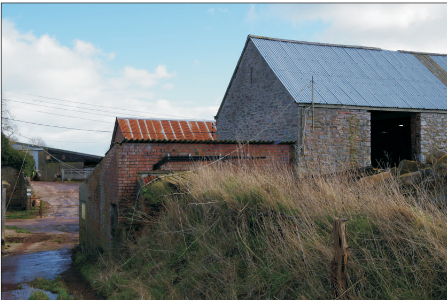
Plate 8: Building 3, southwest elevation (north end) and northwest elevation, showing later extension, viewed from the west.
