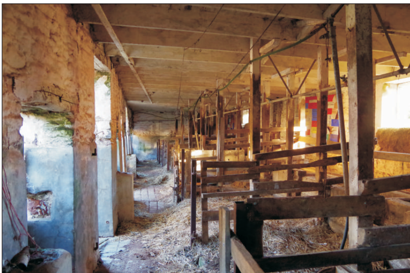
Plate 3: Building 1, interior, viewed from the southeast.
