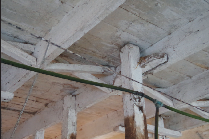
Plate 4: Building 1, detail of the first-floor structure, viewed from the northwest.
