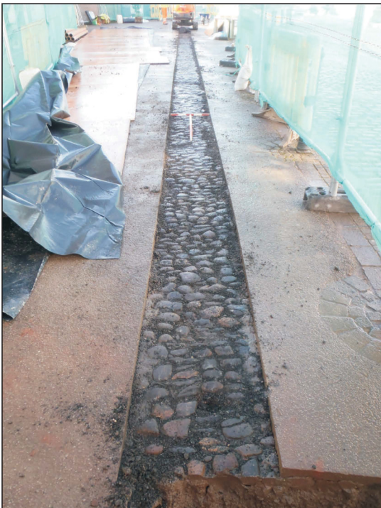
Plate 3: Trench 2, surface F112. 1m and 0.5m scales.
