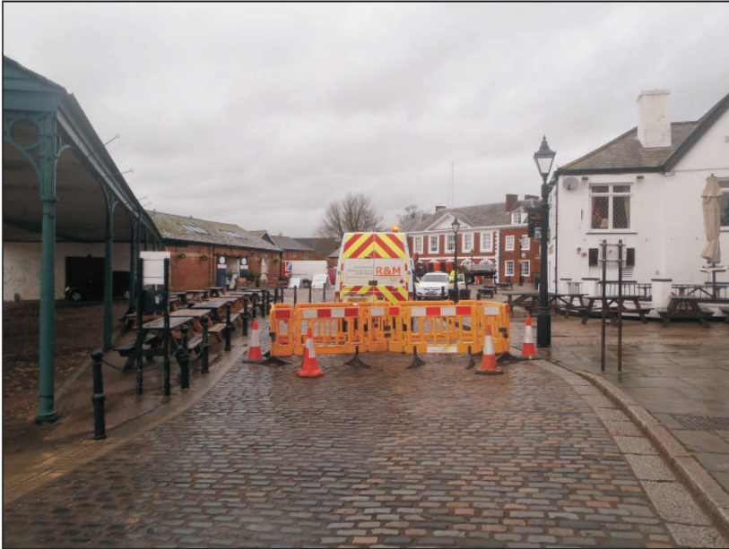
Plate 1: Location of Trench 1 in fenced off area, looking west
