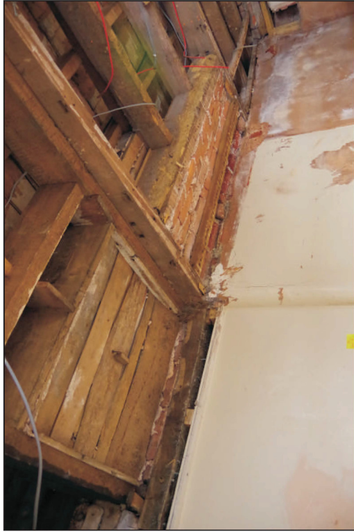
Plate 3: Basement (B4), ceiling with ?hatch and brick fireplace base
