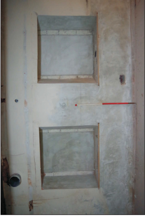
Plate 2: Basement (B3), blocked windows of primary phase west-facing wall (scale 1m)
