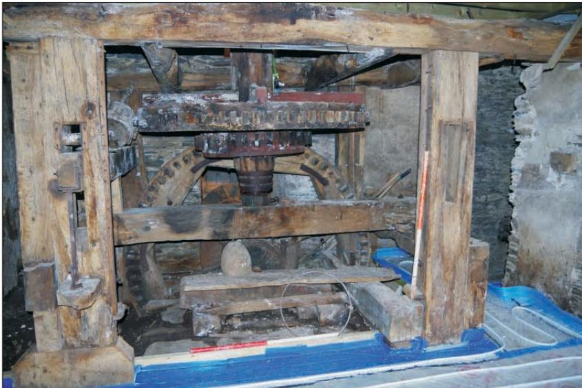
Plate 9: The gears prior to restoration showing the engaging mechanism (and axle) and holes for removed engaging mechanism in the frame, viewed from the west. 2m scales.
