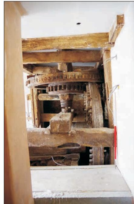
Plate 10: The restored gears showing the pit gear in its pit, viewed from the south. 1m scale.
