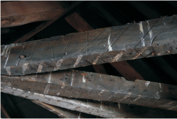
Plate 13: The markings on a roof timber, viewed from the north.
