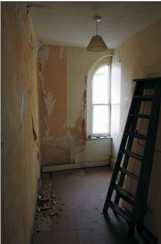
Plate 11: The shared window in bedroom 2, viewed from the south. 1m scale.
