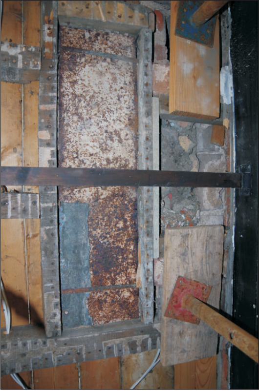
Plate 5: The base of the first-floor hearth looking up from the shop, viewed from the east.
