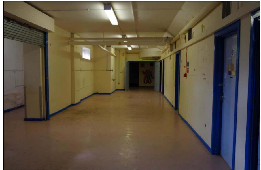
Plate 11: The first floor, looking southwest
