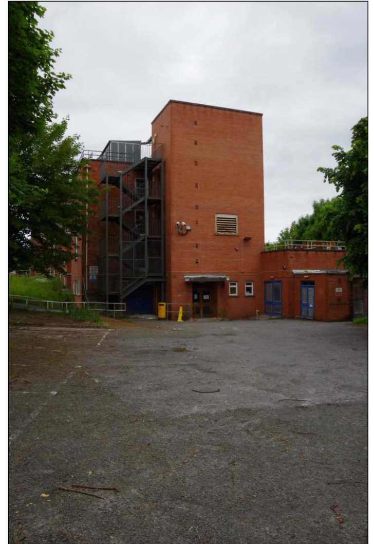
Plate 8: The 1977-78 tower, looking west. 1m scale
