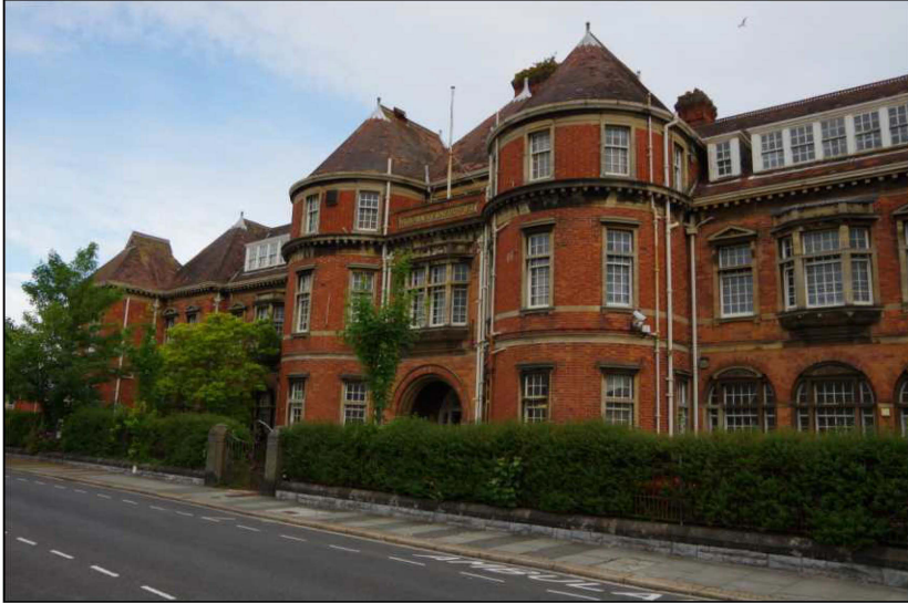
Plate 1: The south front of the original 1901 building, looking northwest
