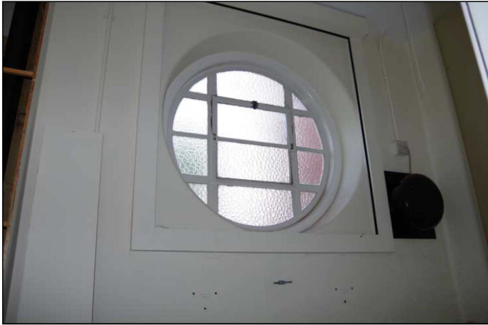
Plate 6: The round window in the north elevation, looking north
