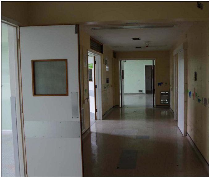
Plate 12: The basement, looking southwest
