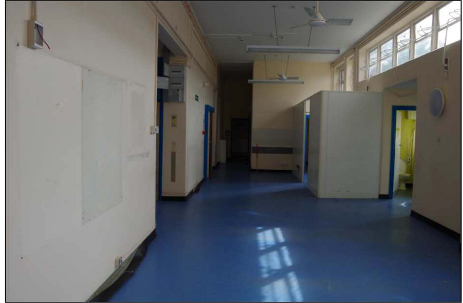
Plate 10: The ground floor, looking northeast. 1m scale
