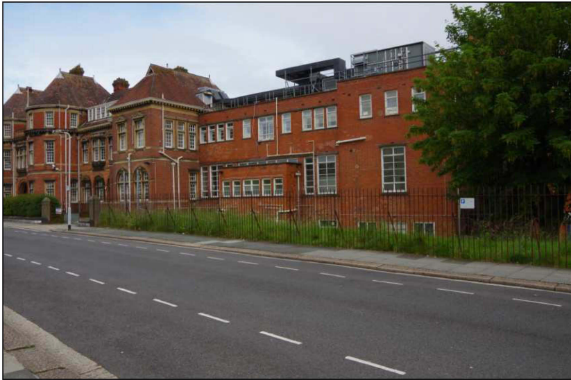
Plate 4: The south elevation of the 1938 extension, looking northwest
