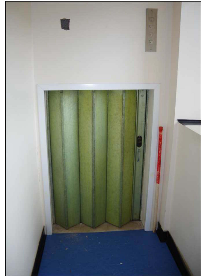
Plate 14: The goods lift, looking northeast. 1m scale
