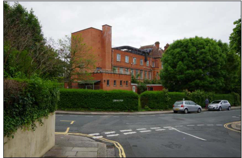
Plate 5: The north elevation of the 1938 extension, with 1970s tower, looking southwest
