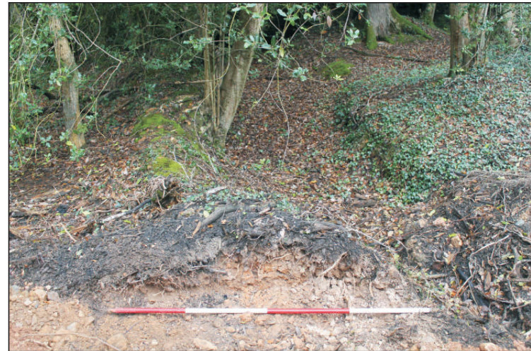
Plate 4: Watching Brief, John Acres Copse, southeast-facing section of Earthwork C (scale 2m)
