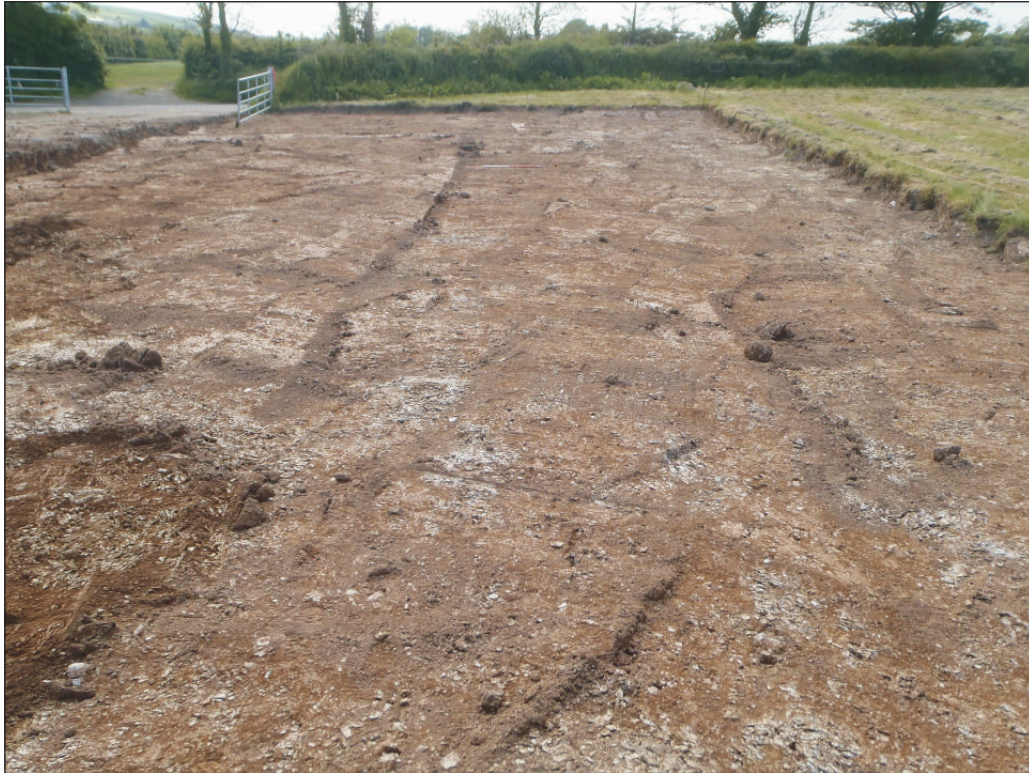
Plate 1: General view of site following stripping, looking west. 1m scale
