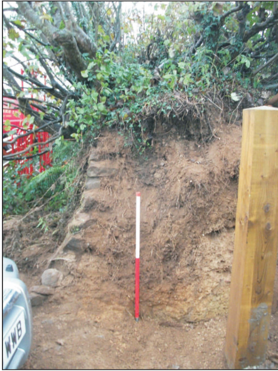
Plate 1: Hedgebank 1, south side, looking west. 1m scale
