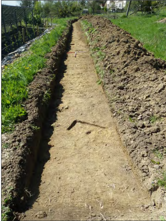
Plate 1: General view along Trench 2, from the east (scales 2 x 1m)
