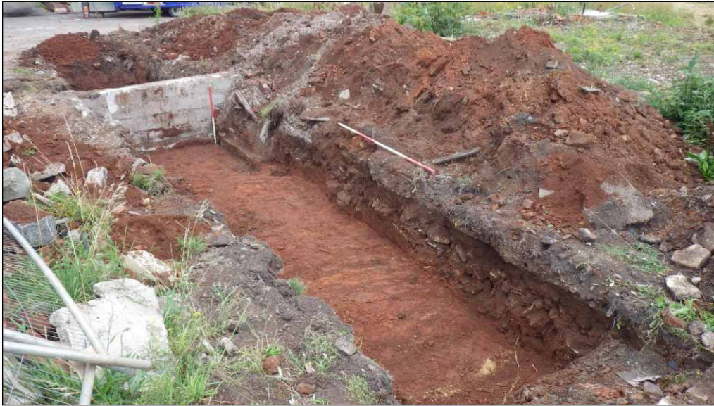
Plate 5: Oblique view of south-west facing section of trench 2 showing footings and construction cuts associated with Granby House, view to the north. 1m and 2m scales
