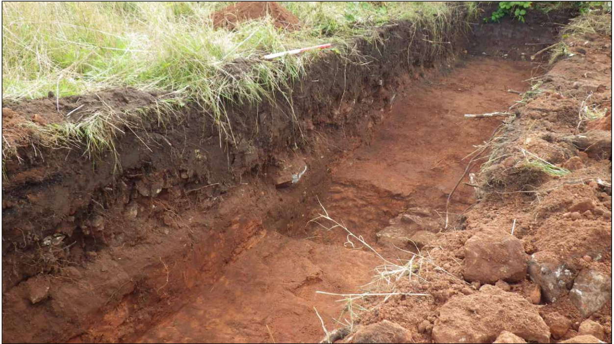
Plate 8: Trench 3, oblique view of south-west facing section showing made ground deposit 301 and F304, view to the east. 1m scale
