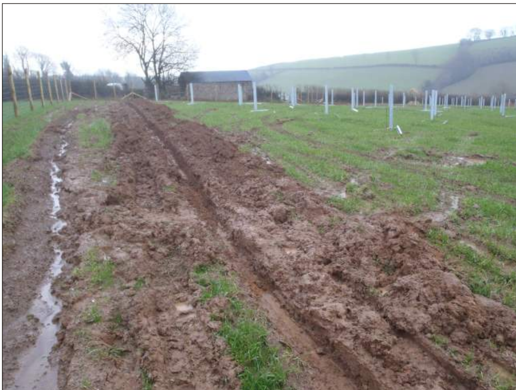
Plate 2: Cable trench, Area 2, looking south-east
