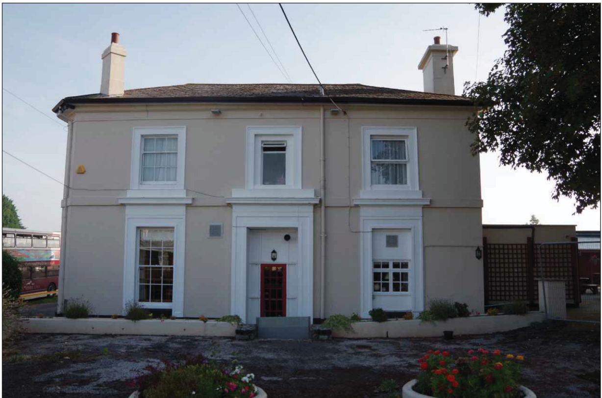
Plate 2: The southwest elevation viewed from the southwest
