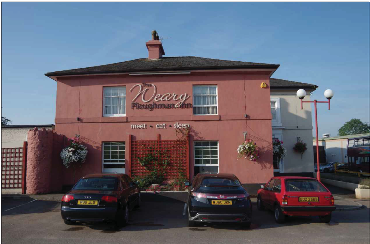
Plate 6: The northeast elevation of the east block showing the gate post to the left viewed from the northeast
