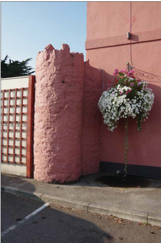
Plate 10: The gate pier viewed from the northeast
