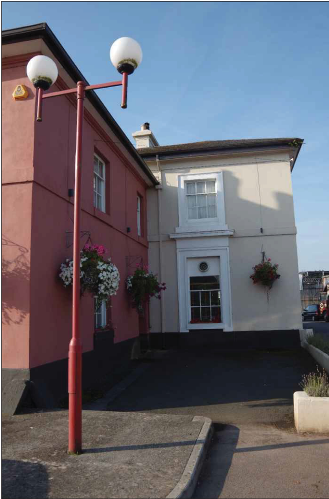
Plate 3: The northeast elevation of the west block viewed from the northeast
