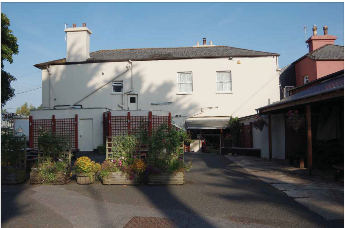
Plate 4: The rear southeast elevation showing the extensions viewed from the southeast
