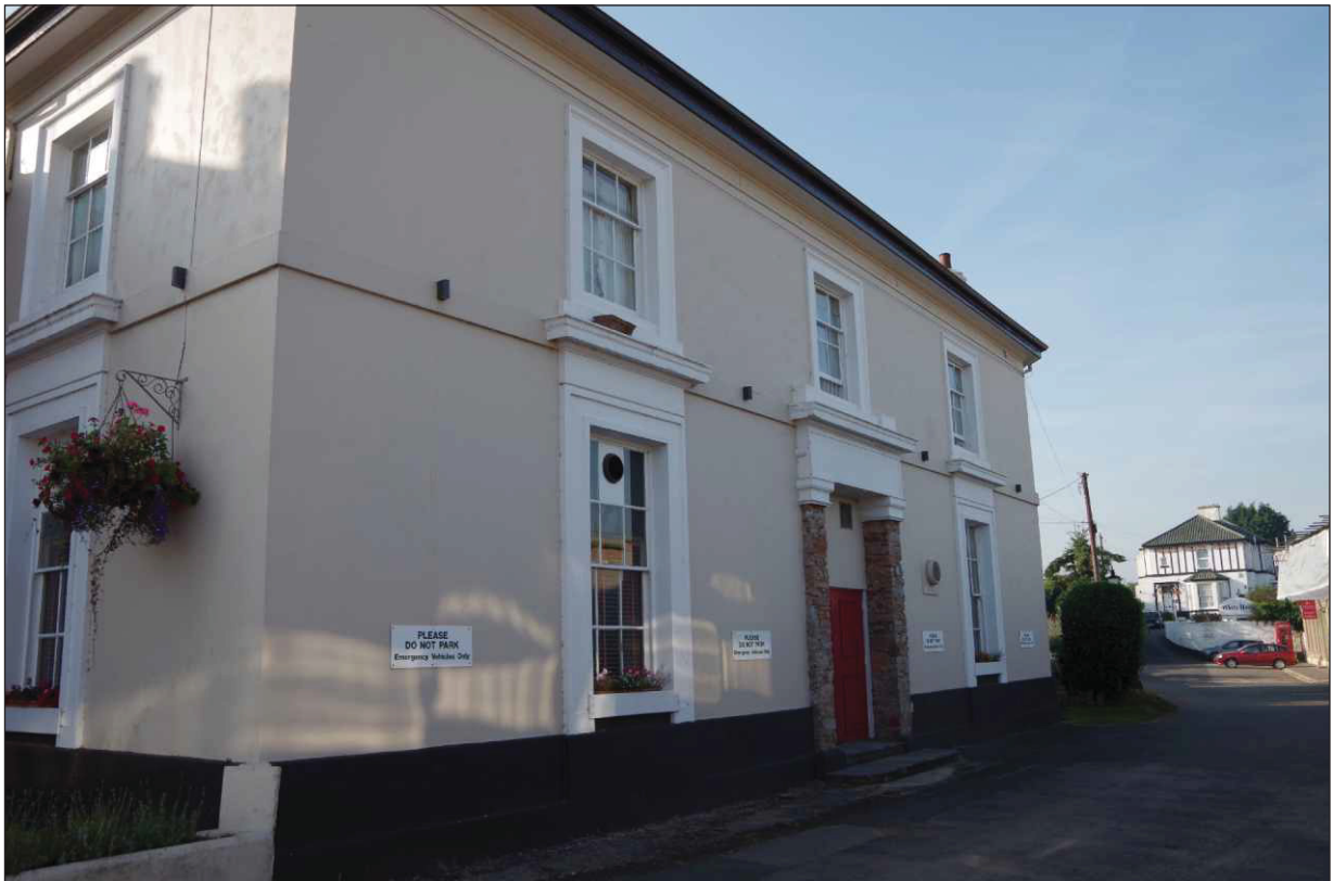
Plate 1: The principal northwest elevation viewed from the north
