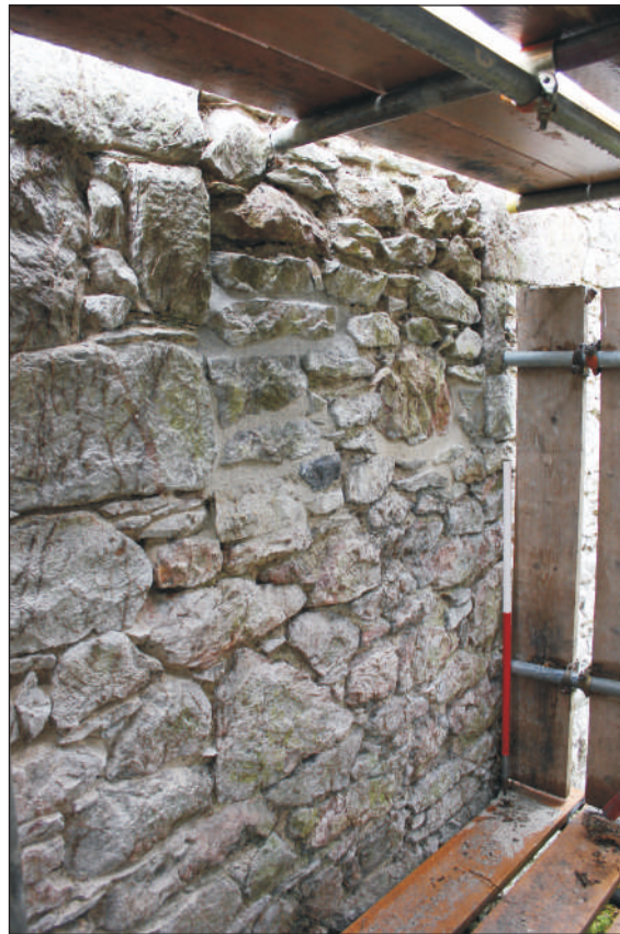
Plate 14: The store, north elevation showing blocked opening, looking southwest. 1m scale.
