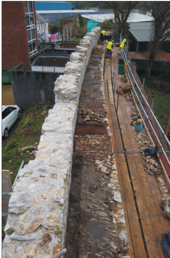
Plate 6: The wall walk during repairs, looking west.
