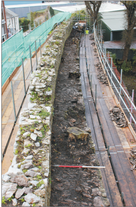
Plate 5: The west end of the wall walk, looking west. 1m scale.
