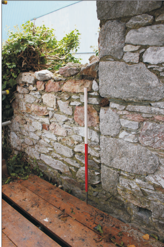
Plate 15: The store, east elevation showing blocked opening and later sockets, looking southwest. 1m scale.
