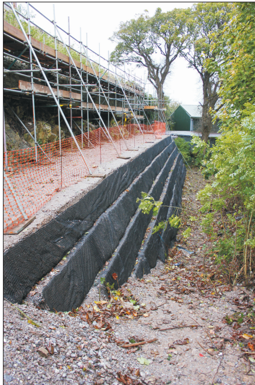
Plate 2: The earth bank supporting the temporary scaffolding, looking southwest.
