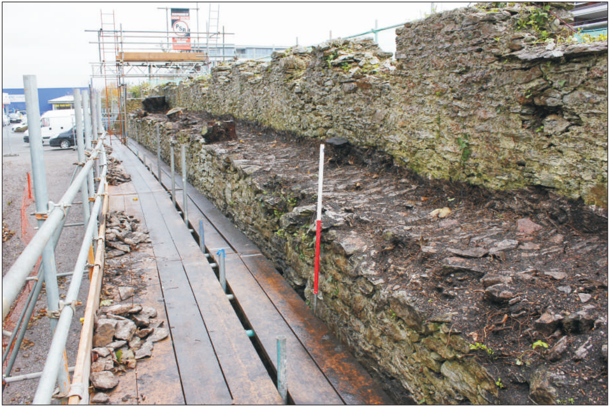
Plate 3: The wall walk following exposure, looking southeast. 1m scale.
