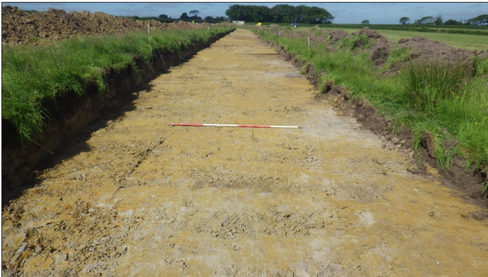
Plate 2: Haul road during stripping looking west. 2m scale.
