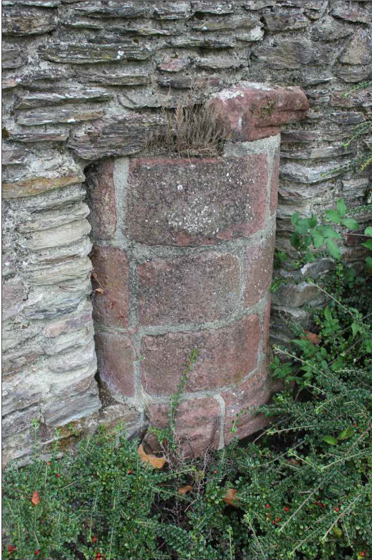
Plate 4: The column rebuilt into the boundary wall of Manor Court
