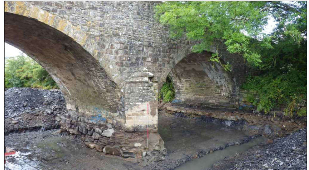
Plate 2: Pier 2 showing pier and cutwater foundations with pier 4 in the background showing foundations laid onto bedrock, viewed from the northeast. Scale 1m
