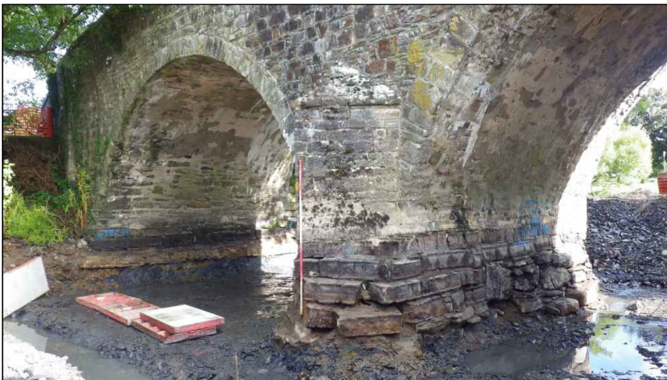
Plate 3: Pier 2 showing stepped cutwater foundations, viewed from the south. Scale 2m
