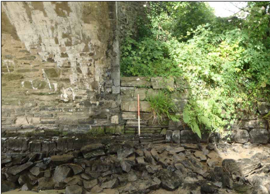
Plate 7: Revetment wall adjacent to pier 4, viewed from the southeast. Scale 1m
