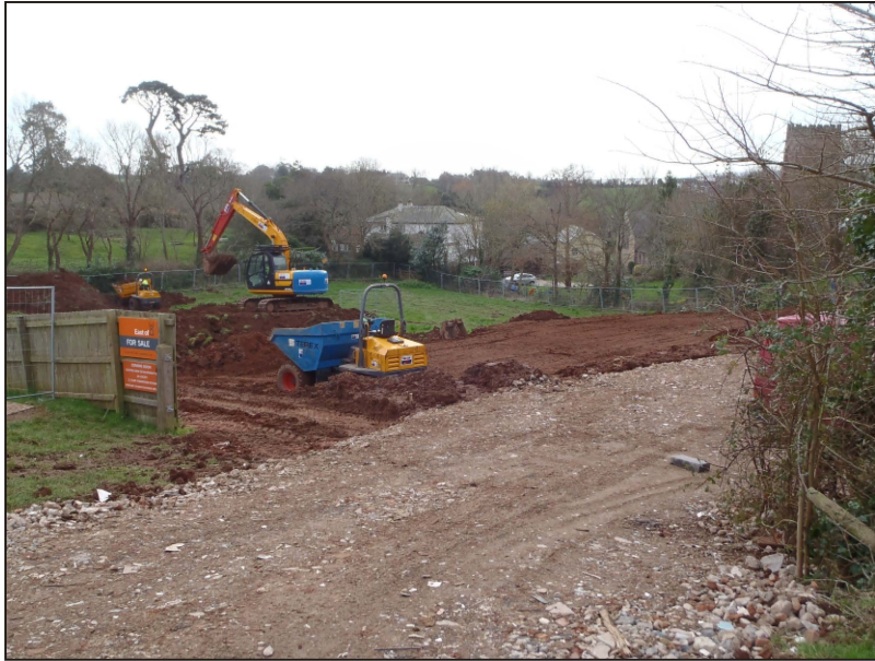
Plate 1: General view of the site, looking south
