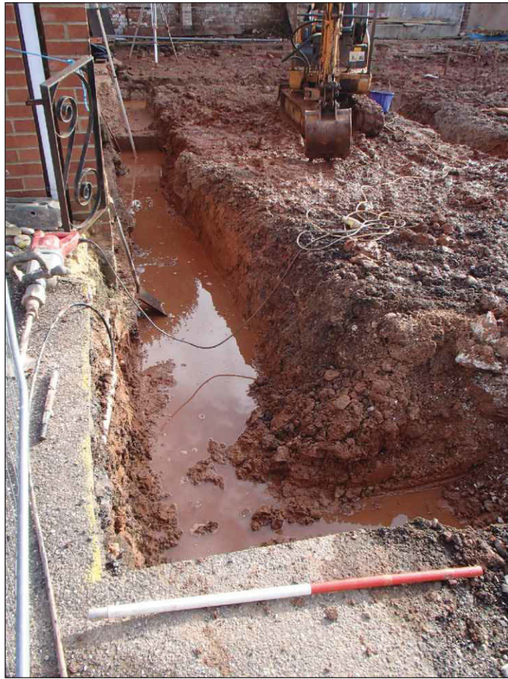
Plate 1: The northern foundation trench, looking east. 1m scale
