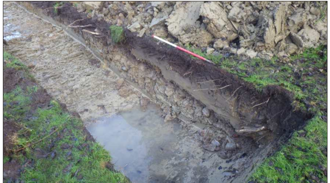
Plate 2: Southwest end of Trench 1, showing demolition layer 101. View to northwest (scale 1m)
