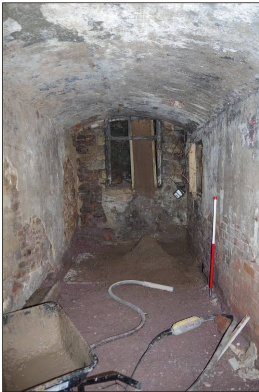
Plate 27: Room LGF8 – barrel-vaulted cellar, looking east. 1m scale
