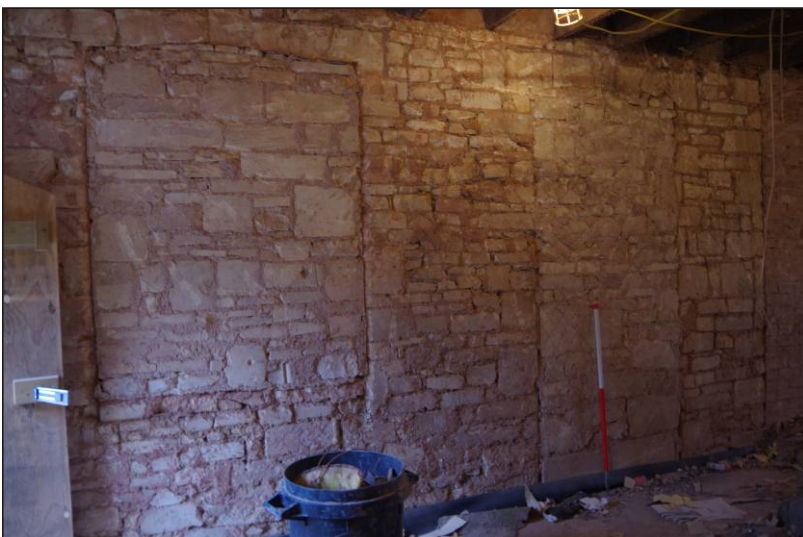
Plate 19: Room GF3 – blocked openings in south elevation, looking southwest. 1m scale
