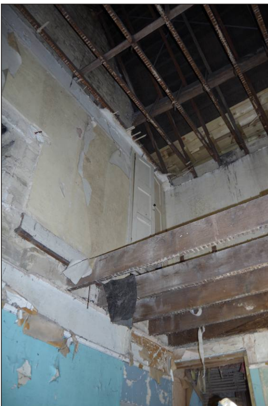
Plate 22: Room FF1 in No. 10 showing cupboards, looking southwest
