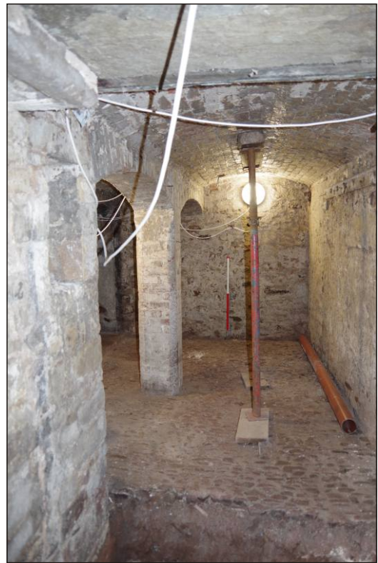
Plate 28: Room LGF10 – barrel-vaulted cellar, looking east. 1m scale
