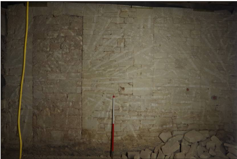
Plate 18: Room GF1 – blocked openings in north elevation, looking north. 1m scale
