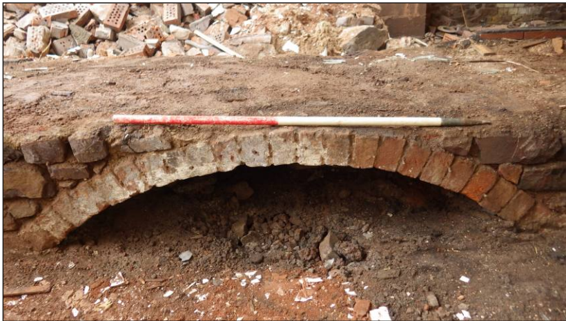
Plate 7: Nos 1 and 2 St Andrew Street, top of cellar arch looking north. 1m scale
