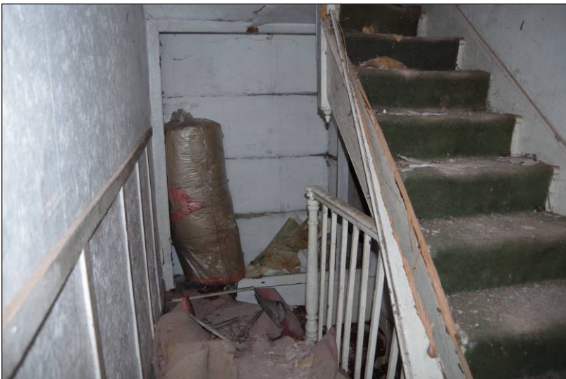
Plate 21: The staircase in No. 9, looking north.
