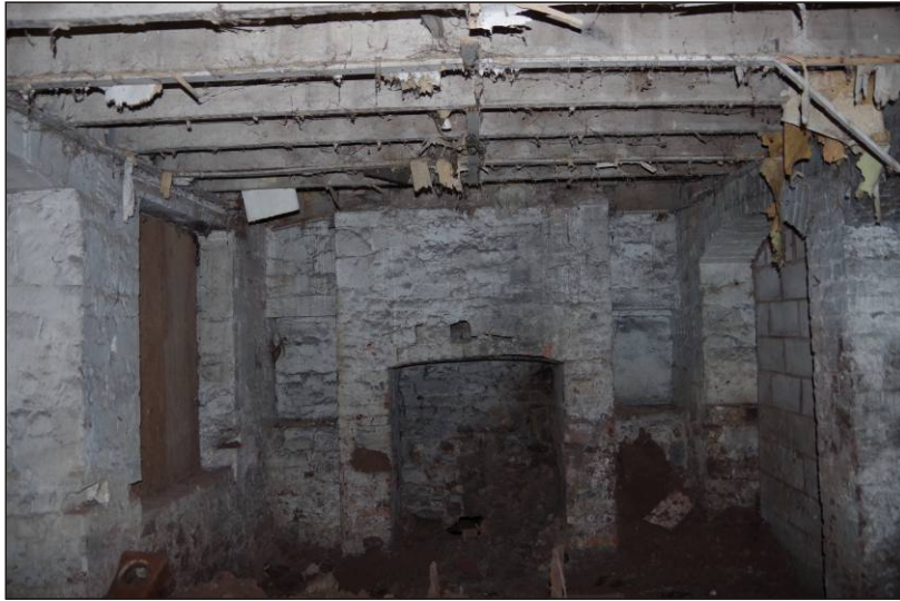
Plate 29: Room LGF11 – basement room showing fireplace and blocked arches, looking west.
