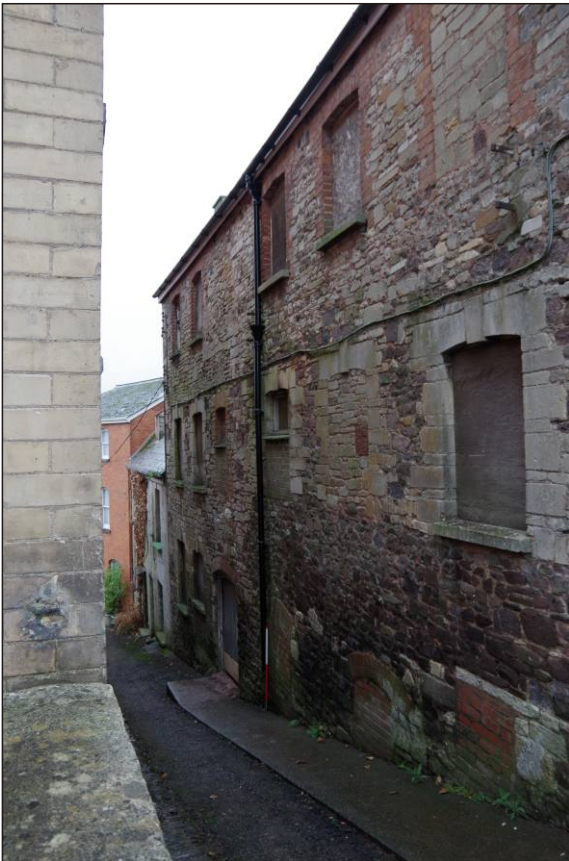
Plate 15: The Ham Place frontage of No. 10, looking northwest. 1m scale
