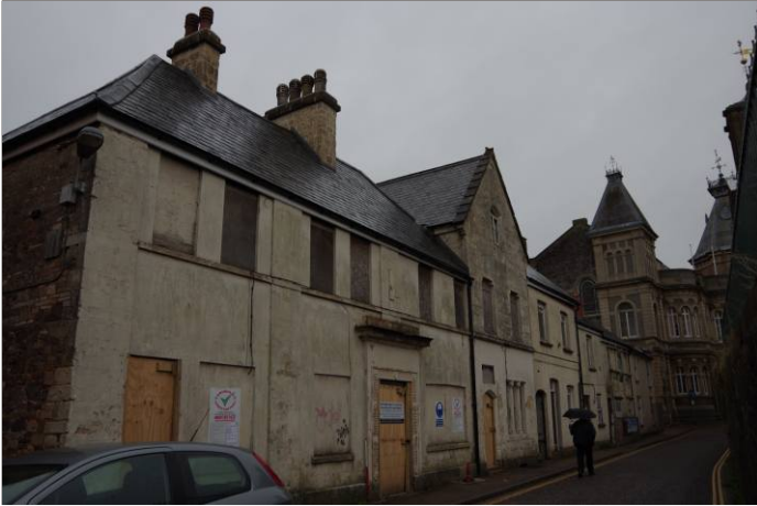
Plate 13: The St Andrew Street frontage looking northwest. 1m scale
