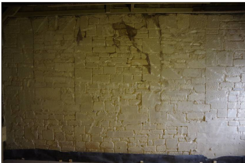
Plate 25: Room FF1 in No. 10 – blocked openings in north elevation, looking north.
