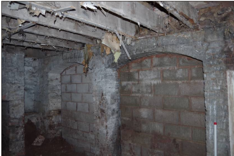
Plate 30: Room LGF11 – basement room showing blocked arches, looking northwest.
