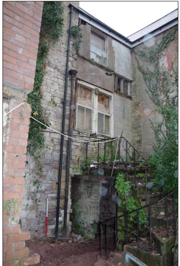
Plate 16: The northwest corner of No. 10, looking southeast. 1m scale
