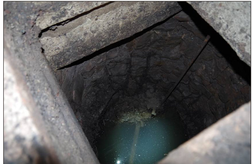
Plate 12: Well in No. 10 St Andrew Street, looking northwest.
