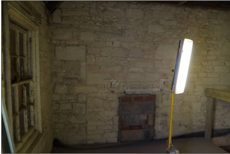
Plate 23: Room FF1 in No. 10 – blocked opening east of fireplace, looking south.
