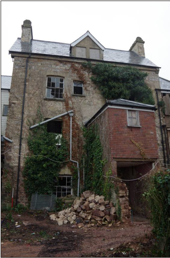
Plate 17: The west elevation of No. 9, looking east. 1m scale
