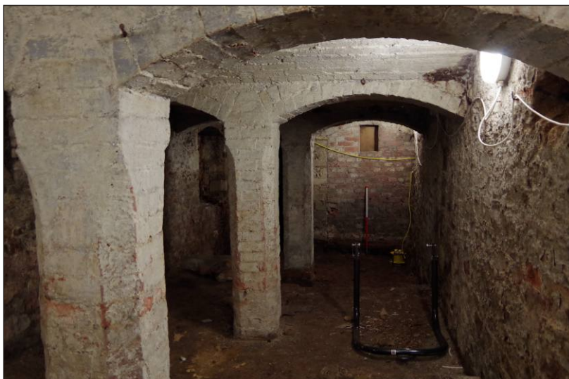
Plate 31: Room LGF12 – barrel-vaulted cellar, looking east. 1m scale
