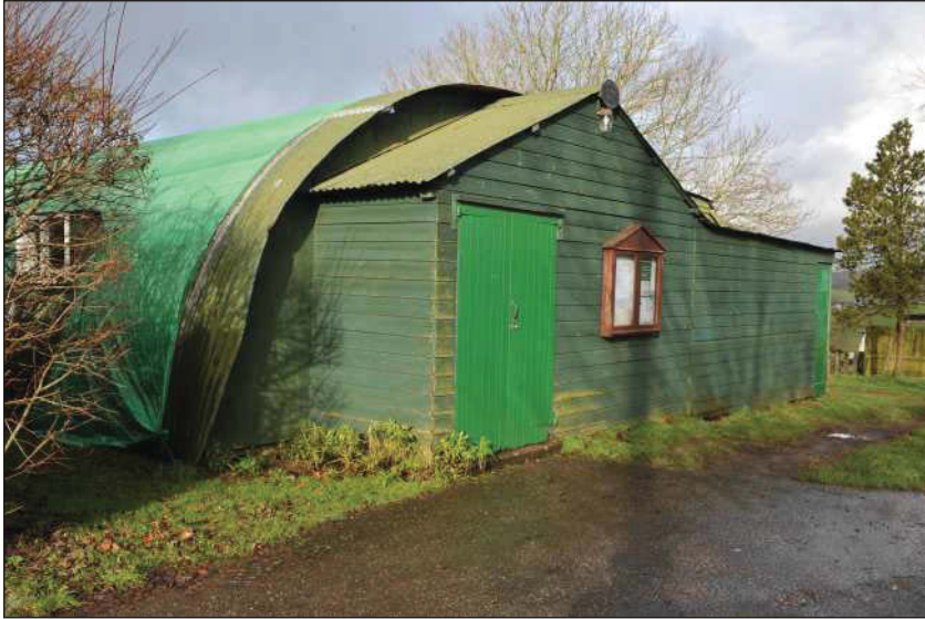
Plate 9: The lobby, viewed from the south.
