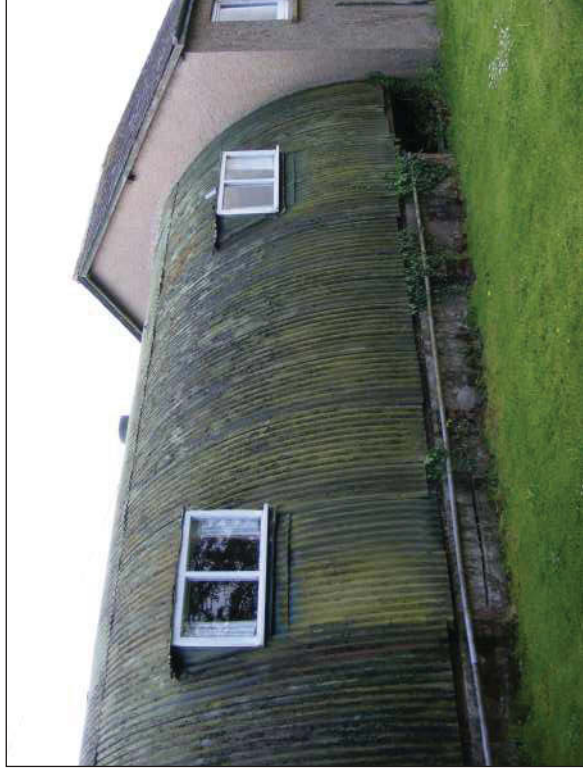
Plate 6: The north side of the hall showing the corrugated iron covering and windows, viewed from the northeast. Photograph © Mike Passmore
