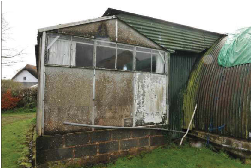
Plate 10: The west elevation of the bar/store extension, viewed from the northwest.
