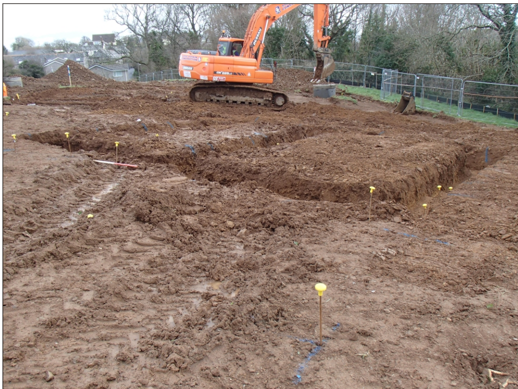
Plate 2: Foundations digging, looking east
