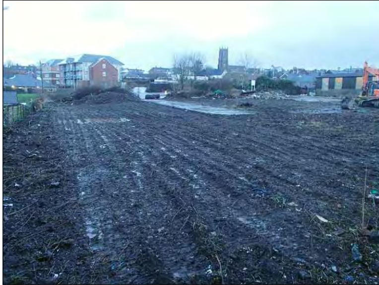
Plate 1: General view of site, looking northeast
