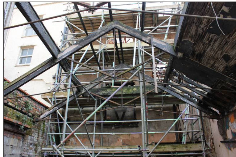
Plate 19: The roof structure of the rear outbuilding, viewed from the northwest.
