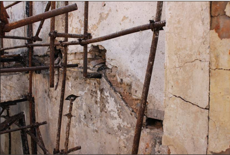
Plate 8: The chase for the stairs to the rear first-floor door, viewed from the north.
