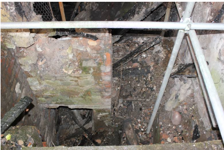
Plate 15: The possible rear entrance to the basement, viewed from the northwest.
