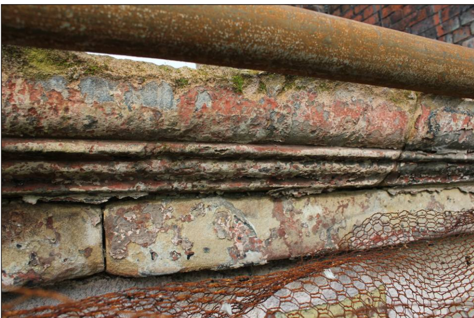
Plate 6: Detail of the cornice at eaves level, viewed from the southeast.
