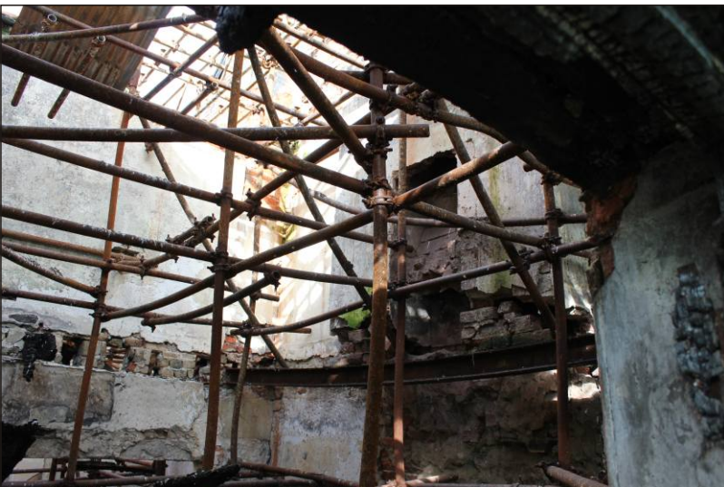
Plate 9: The first-floor fireplace in the front room, viewed from the south.
