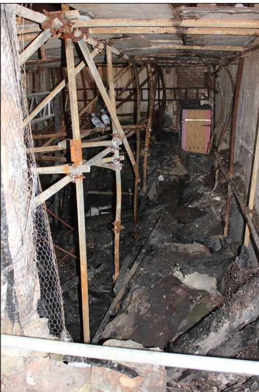
Plate 12: The ground-floor looking southeast along the line of the possible corridor.
