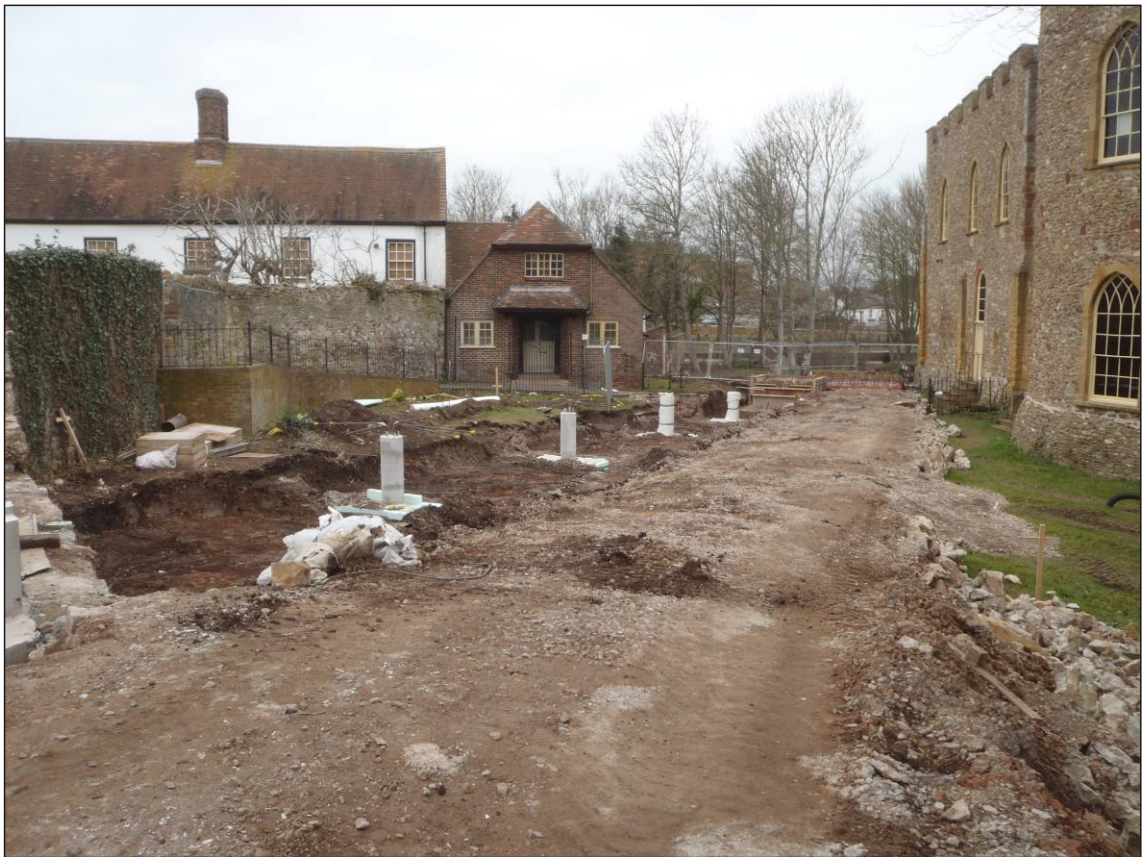
Plate 14: Work in progress for footbridge construction, looking northwest
