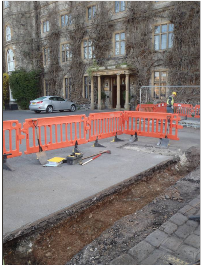
Plate 8: Excavation Area 3, excavation in progress, looking northeast (scale 1m)
