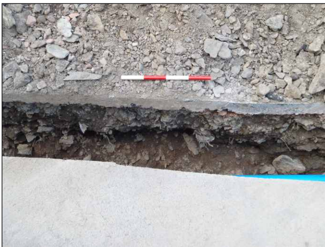
Plate 2: Northeast facing section of the pavement trench, scale 0.50m
