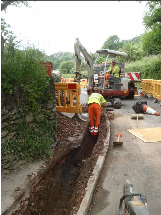
Plate 1: Working view of pavement trench from the southeast
