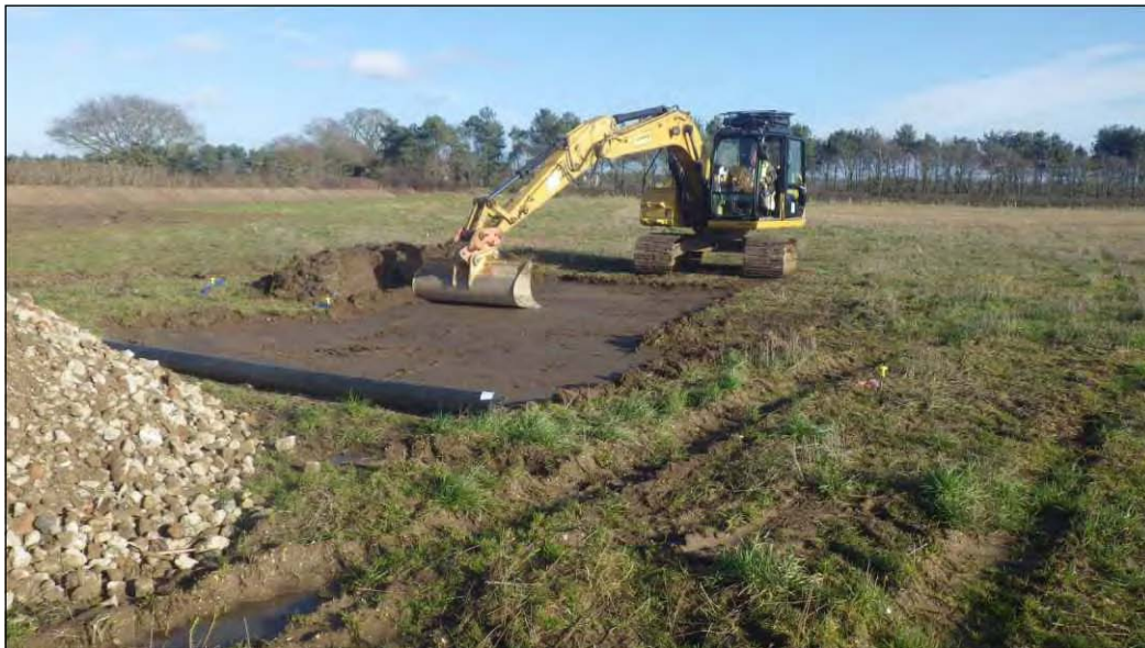
Plate 3: General view of topsoil stripping for a haul road, looking northeast
