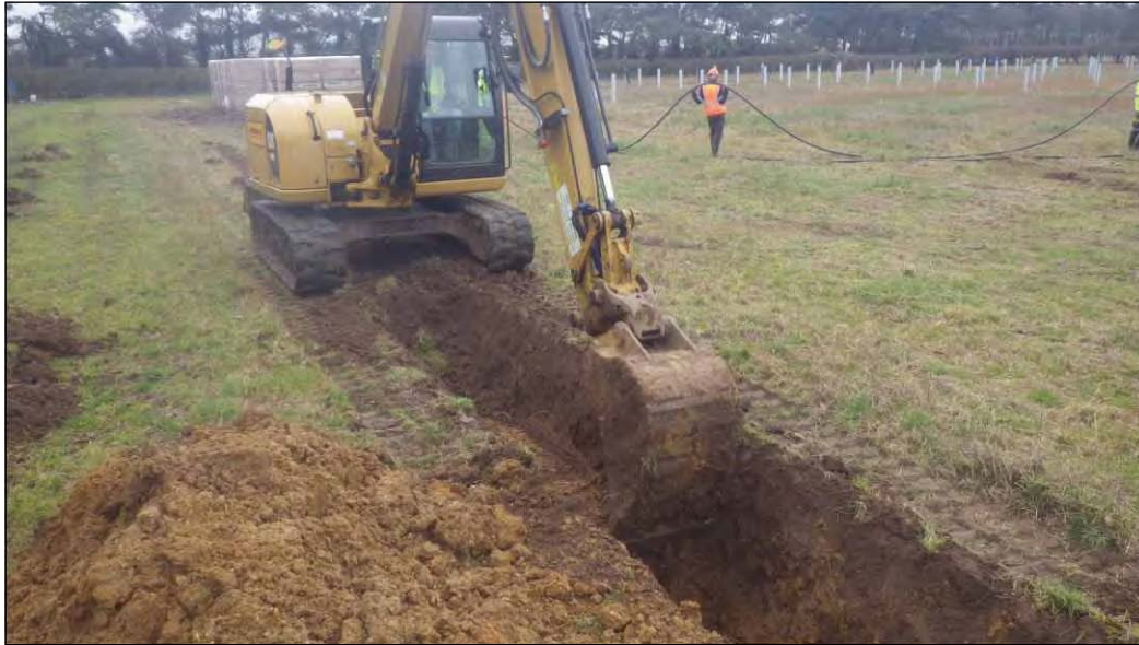
Plate 1: General view of the cable trench excavations, looking southwest
