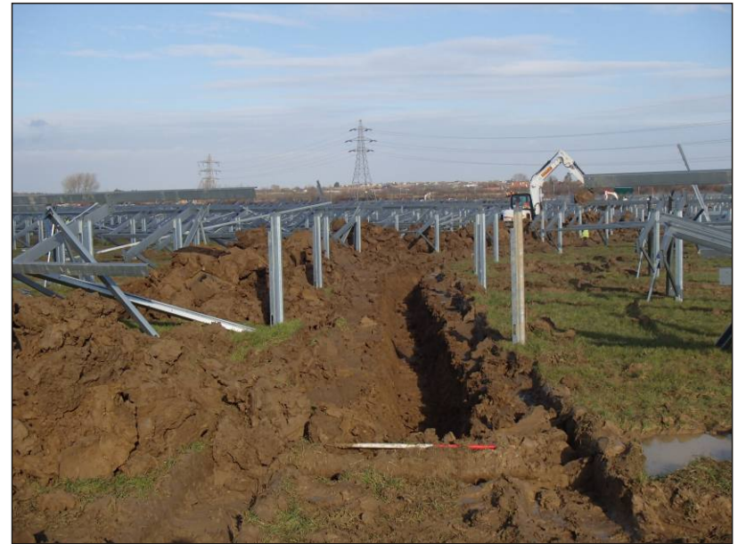
Plate 2: Field 7, general view showing a cable trench, looking northwest
