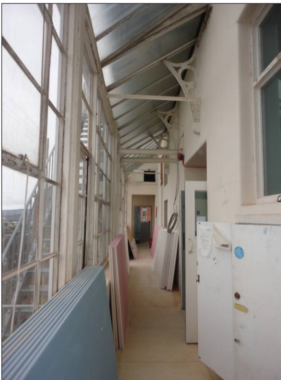
Plate 14: Halford Wing, second floor, sun lobby
