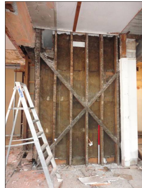
Plate 4: Dean Clarke House, first floor, former central ward, exposed partition
