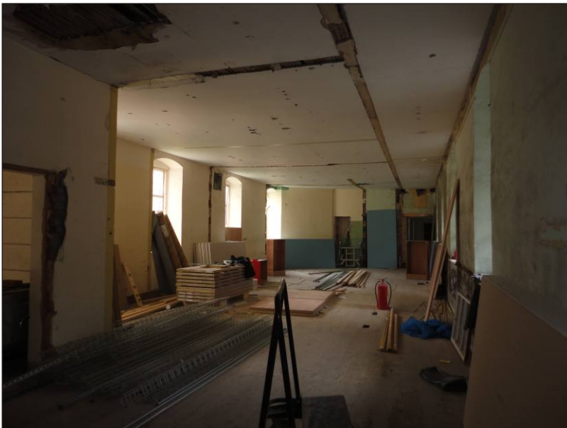
Plate 3: Dean Clarke House, ground floor, former women's ward
