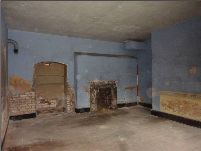
Plate 16: Halford Wing, basement, fireplace
