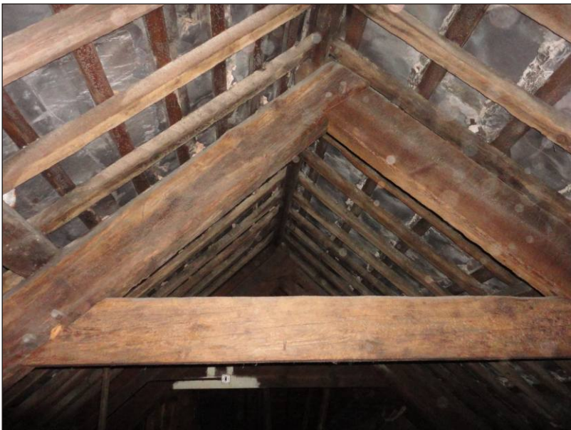
Plate 7: Dean Clarke House, south wing extension, roof space detail
